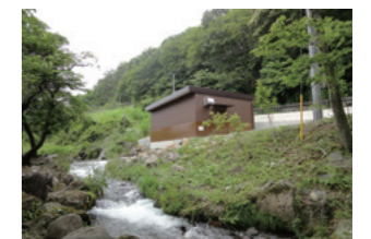
Micro-scale hydro-power station (Hokuto City, Yamanashi Prefecture)
