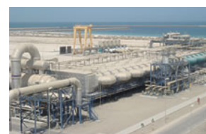
Taweelah B Power & Desalination Complex
