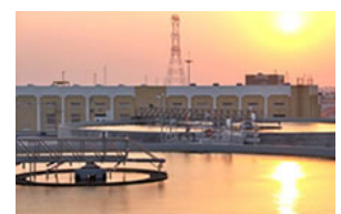
Doha West sewage treatment plant
