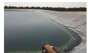
Lusail sewage treatment plant
