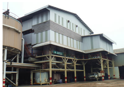
Factory exterior (partial)
