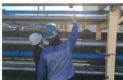
On-site inspection in progress
