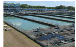
Maynilad water purification plant
