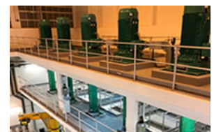
Lusail sewage treatment plant
