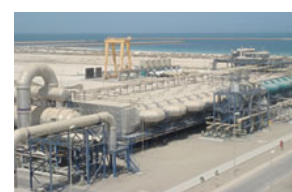
Taweelah B Power & Desalination Complex
