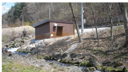
Micro-scale hydro-power station (Hokuto City, Yamanashi Prefecture)
