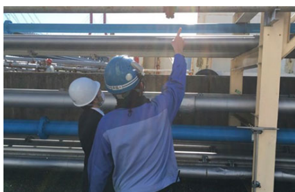
On-site inspection in progress
