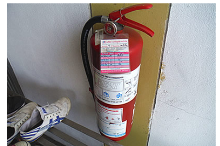
An inspected fire extinguisher
