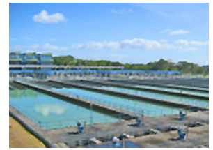
Maynilad Water purification plant
