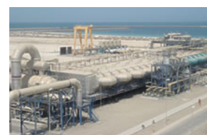
Taweelah B Power & Desalination Complex
