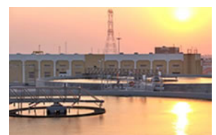
Doha West sewage treatment plant
