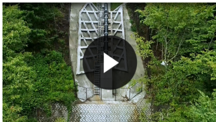
Producing power locally: Mibugawa Power Company
