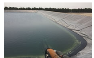
Lusail sewage treatment plant
