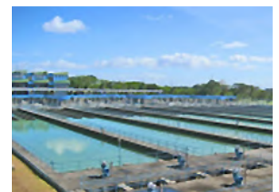
Maynilad Water purification plant
