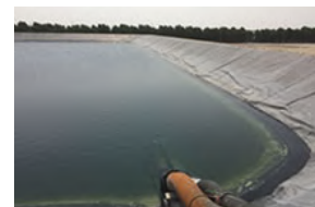
Lusail sewage treatment plant
