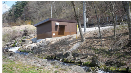
Small hydropower station (Hokuto City, Yamanashi Prefecture)
