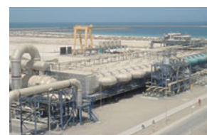
Taweelah B Power & Desalination Complex
